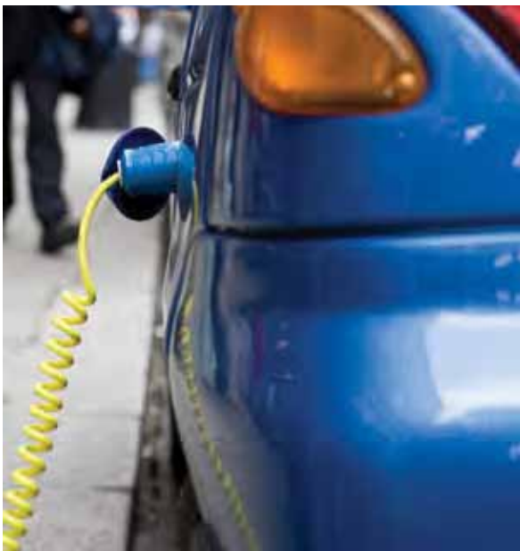
The Government is offering up to £30 million to help install electric vehicle charging points
