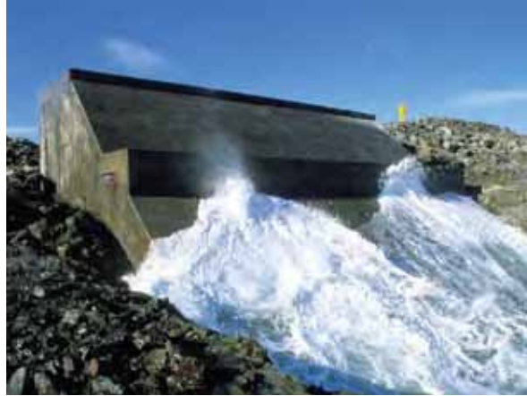
Wave striking Limpet 500, the world's first commercial-scale wave power station. Limpet generates 500 kilowatts of electricity, enough to power 300 homes (Islay, Scotland)
