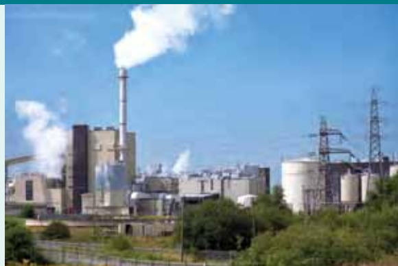
Shotton paper mill is saving CO 2 with a biomass Combined Heat and Power plant
