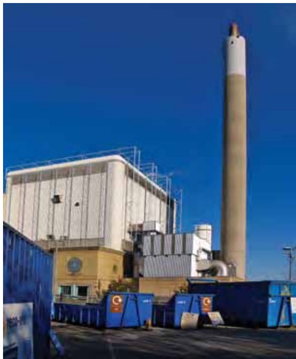
CHP facility in Lewisham, South East London Businesses are exempted from climate change Levy for good-quality combined heat and power plant
